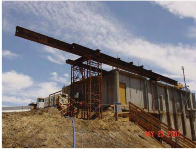
Figure 1. Temporary support of an existing structure
