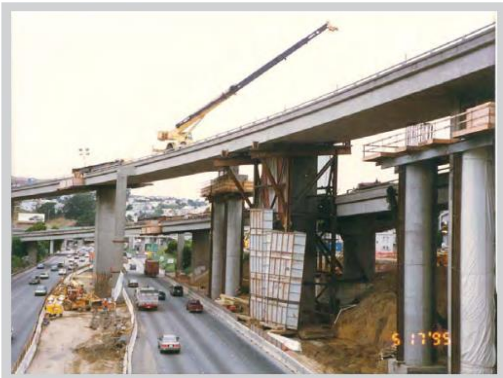
Figure 15. Highway 280 split going over Highway 101 in San Francisco.
